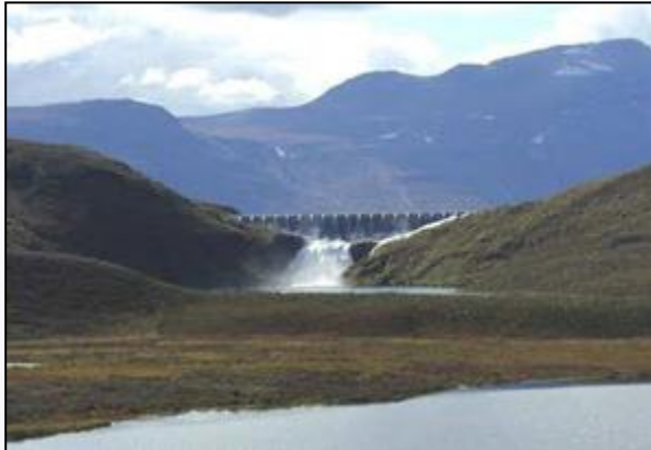
Buksefjord Hydroelectric Station - Greenland
