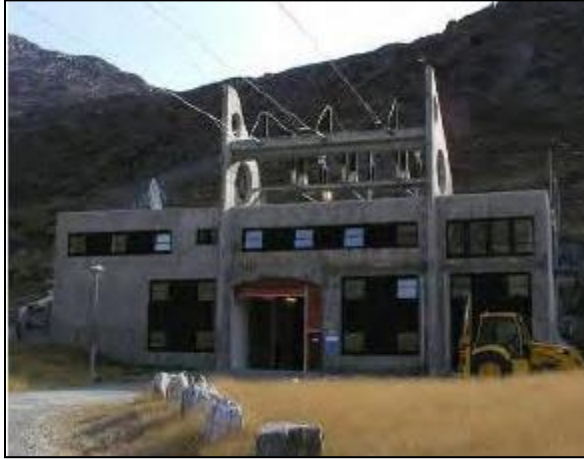
Buksefjord Hydroelectric Station - Greenland
