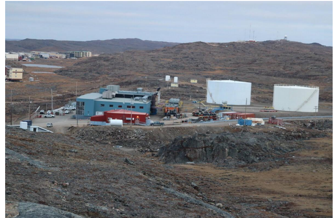
Qulliq Energy Diesel Power Generating Station, Iqaluit
