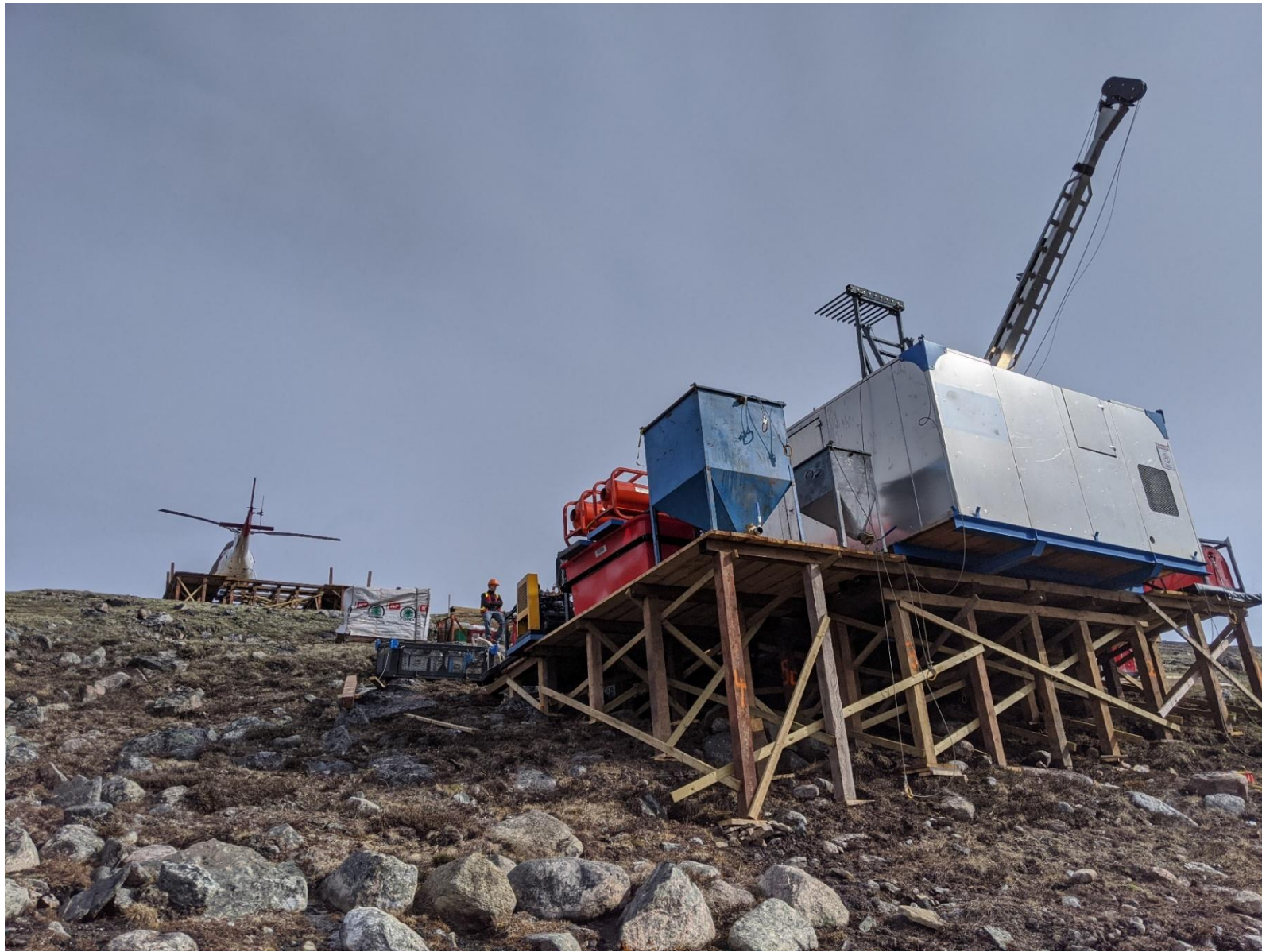
Drill at Western end of Deposit 3
