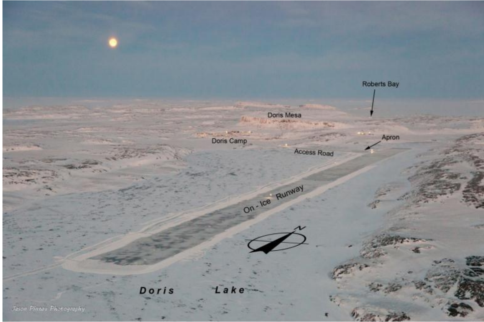
Photo B-1: Runway under construction, December 12, 2011.
