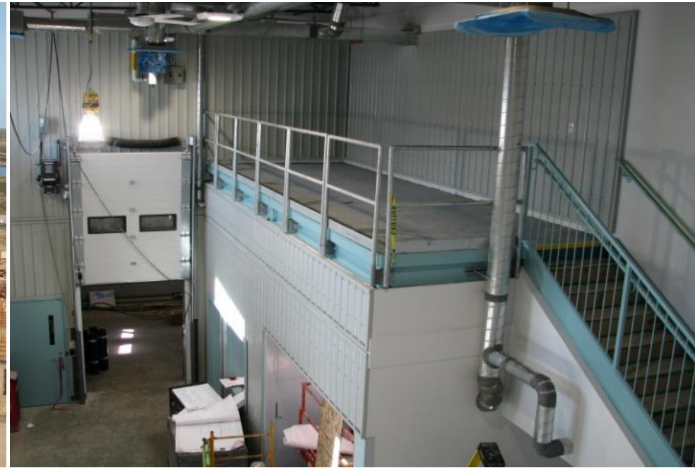
Interior of the Field and Maintenance Building
