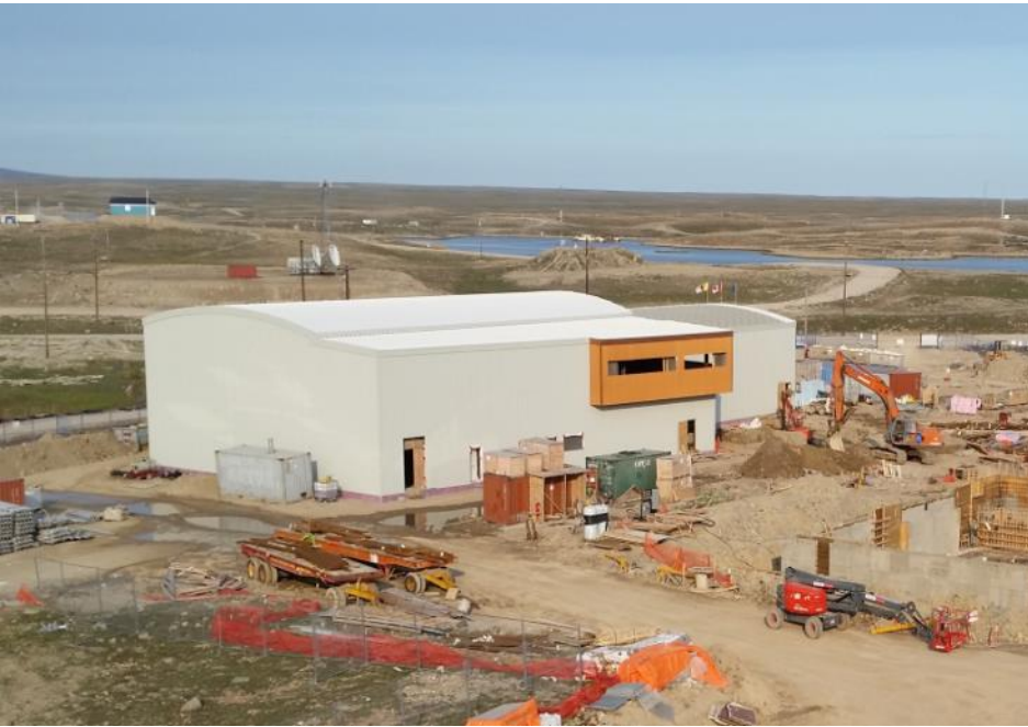
Exterior of the Field and Maintenance Building
