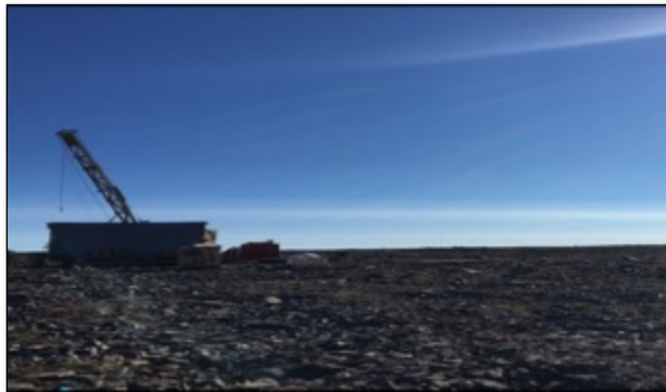
Drill Rig at CH-6
