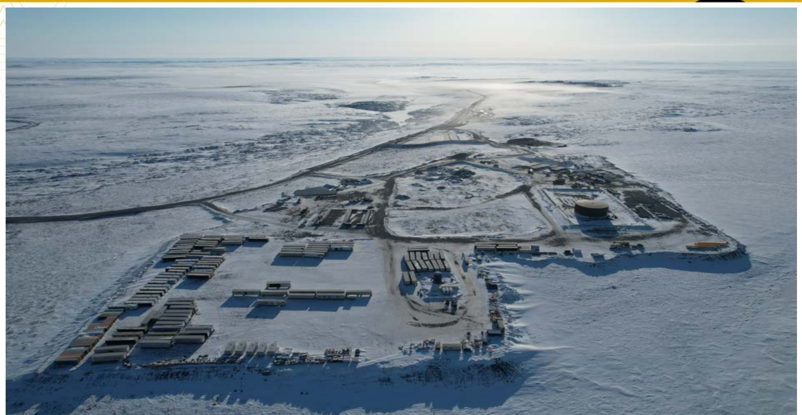
Goose Camp and Plant Site Pads, April 2023
